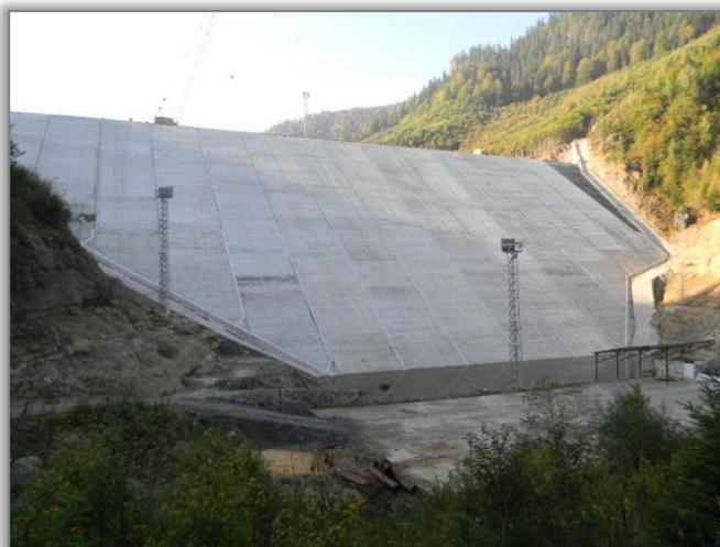
Răstolița Dam – The upstream - Mask concrete
