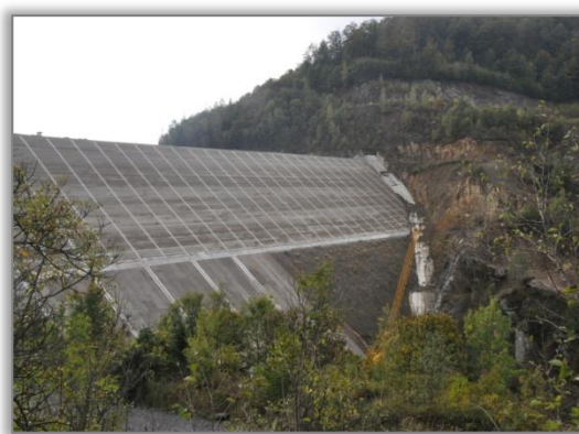
Runcu Dam – upstream sealing mask
