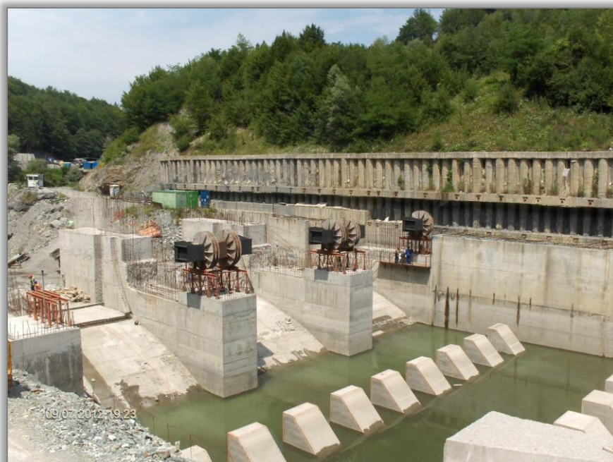
Livezeni Dam– view of to the downstream energy dissipater
