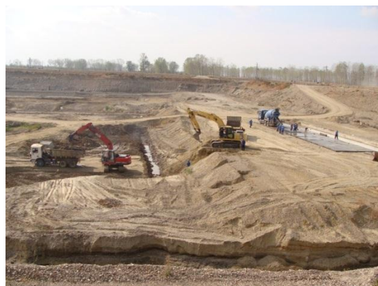
Costesti hydraulic node - Concrete slab dam leveling
